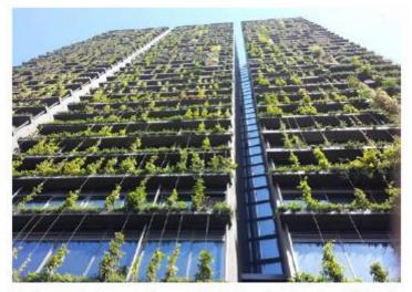
**Photo 4.15a** Planting can be integrated into the facade design, via sophisticated detailing and consideration of ongoing care and maintenance required.
